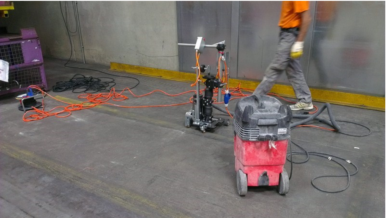
preparing the pouring of new magnesit screed
