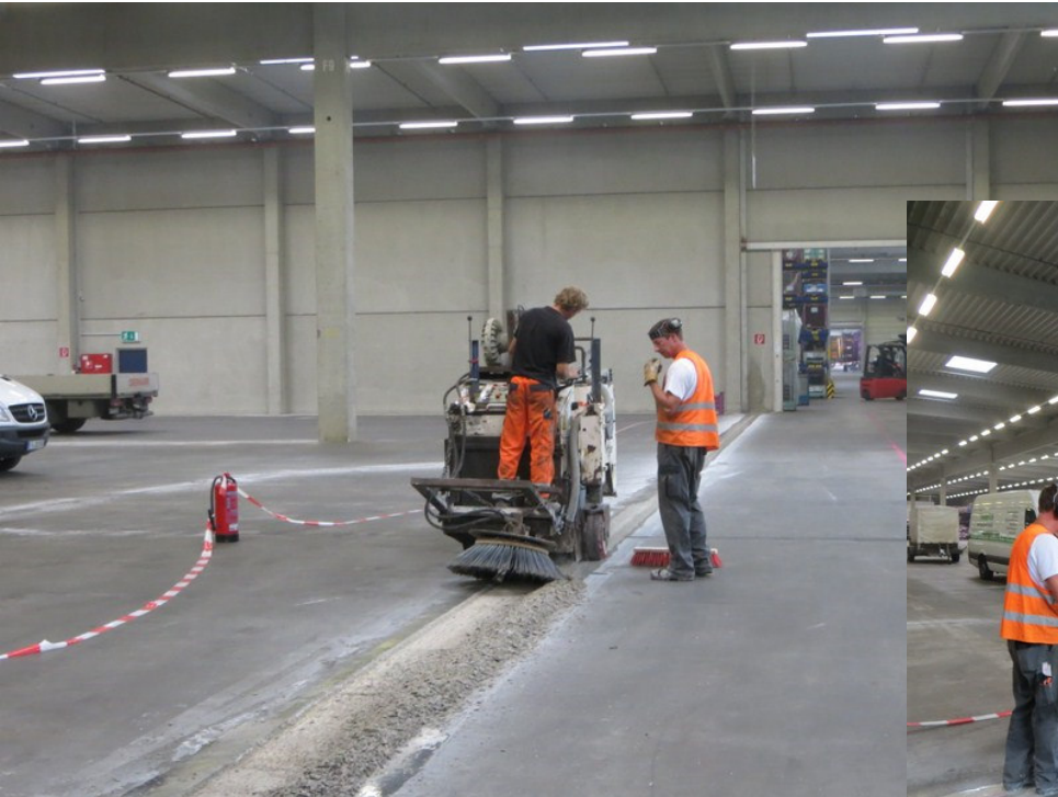
preparing the pouring of new magnesit screed
