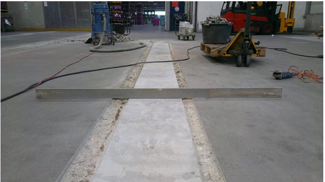
Repair of the existing slabs
