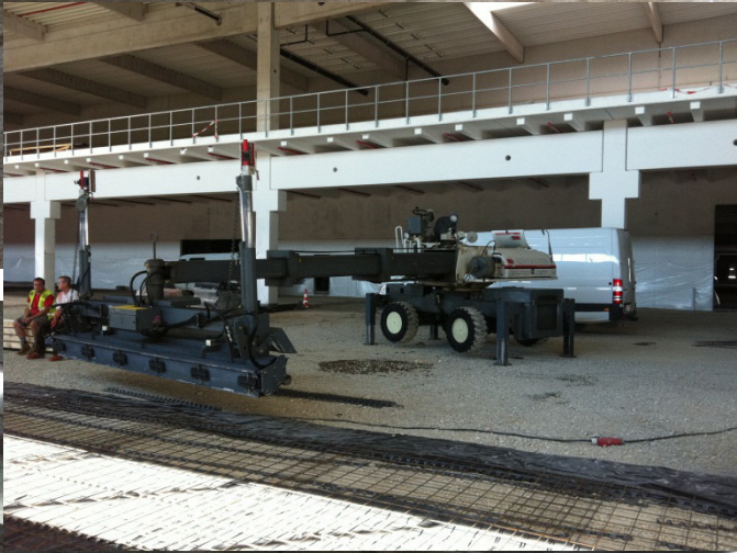
Pouring with Somero SXP Laserscreed
